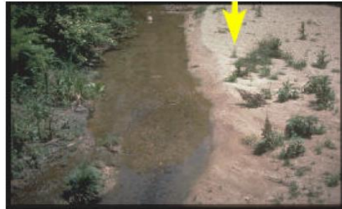
Poor Range (arrow pointing to streambank with almost no vegetative cover)
