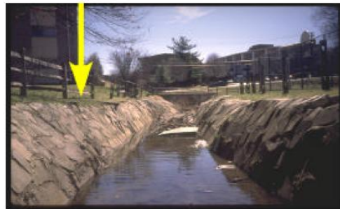
Poor Range (arrow pointing to channelized streambank with no vegetative cover) (MD Save Our Streams)
